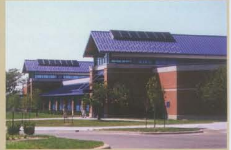
In Kansas City, Casey and Associates converted an abandoned grocery store into a state of the art data center for Jack Henry & Associates of Monett.
